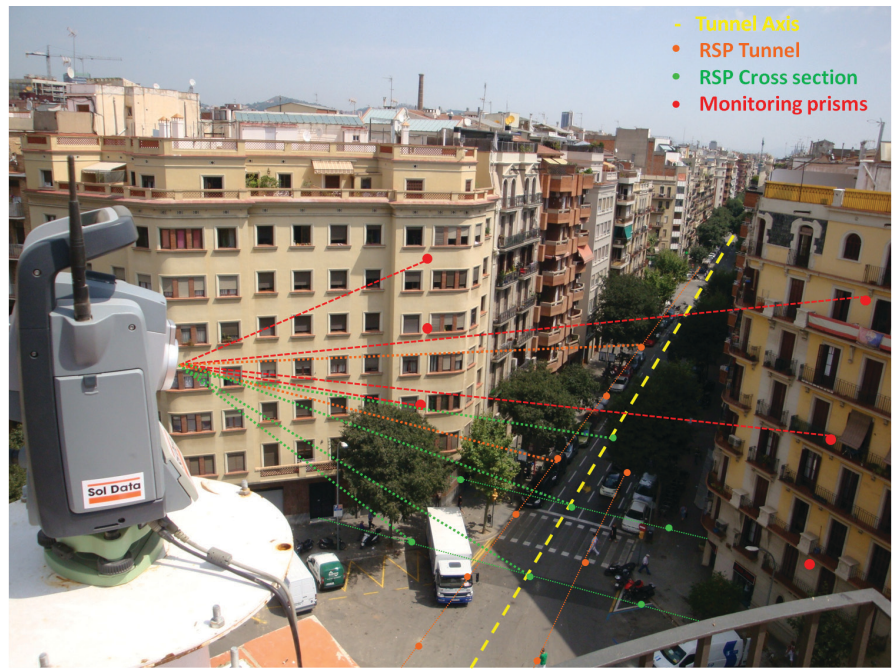
Figure 1. Example of Reflectorless Robotic Total Station (RRTS) installation able to measure RSPs and prisms.
